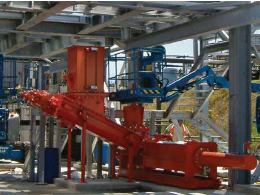
3 Piston pump for feeding pasty solids to co-processing
